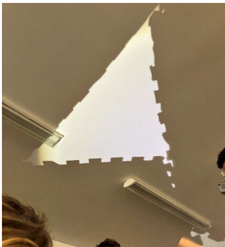
Figure 13: Hawkins|Brown Steam Lab: A new space in the ceiling opens up.
